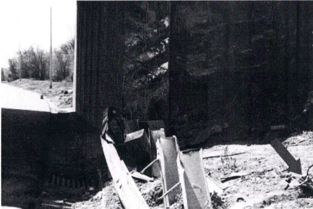
Figure 12. Guardrail damage, light pole base (indicated by arrow), and bridge abutment scrapes.
